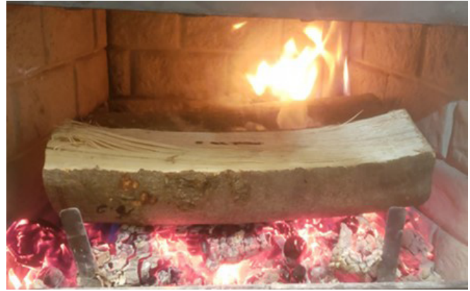
Figure 25: Maintenance-fire load in firebox
