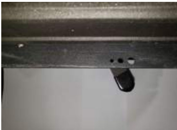
High fire air control (max. position)
