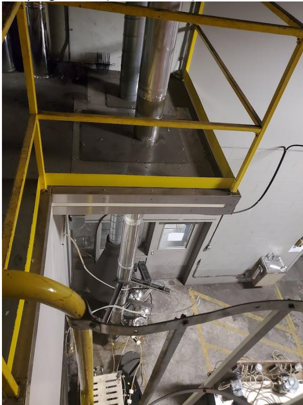
Sampling Section (elbow to floor)
