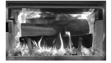
Close the primary air control by small increments (ex: 1/16 of an inch), from ½" to fully closed, between 4 and 15 minutes after the loading period. Before closing further, make sure the flame intensity is increasing or stable. Close the air control completely. Turn ON the blower at maximum speed.
