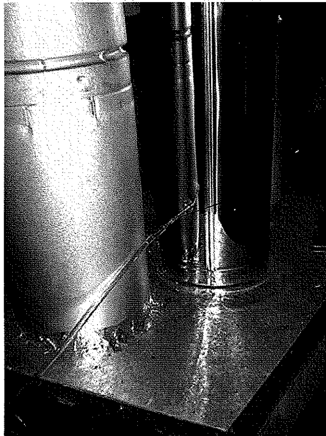
Draft sampling port located 6 in. from flue outlet
