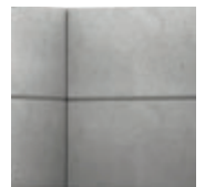
Moulded brick panels – contemporary
